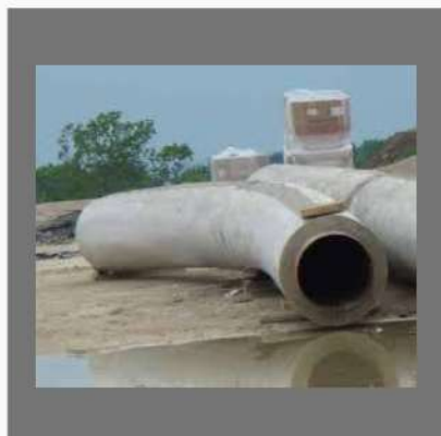
Concrete Pipe Line Bend
