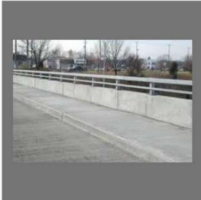
Highway Bridge Parapets (railing)
