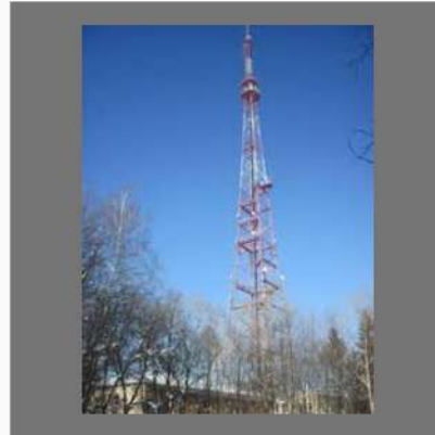
Tv. Transmission Towers (heavy & Light)
